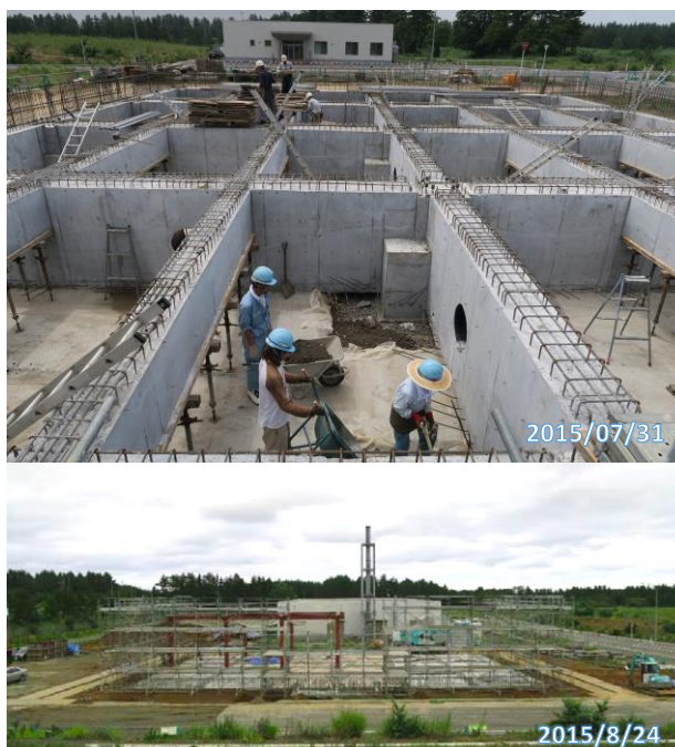
Fig. 2 Current status of the construction of the DEMO Joint Research Building
