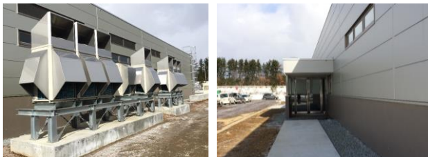
Fig. 1 Exterior views of the DEMO Joint Research Building
