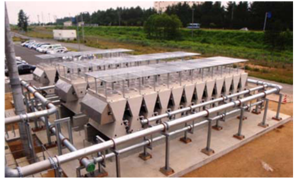
Chiller units with snow protection; photographed on 19/July/2011
