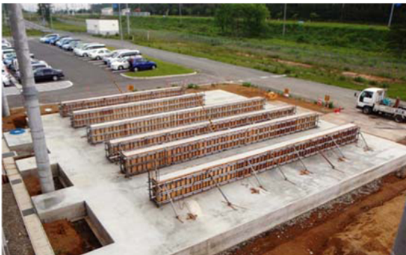
Foundations for chiller units for the supercomputer; photographed on 22/June/2011
