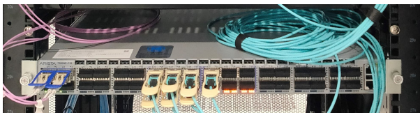
Fig-1 The new 100Gbps network switch (bottom)
